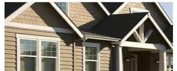
Example: Cementitious material
